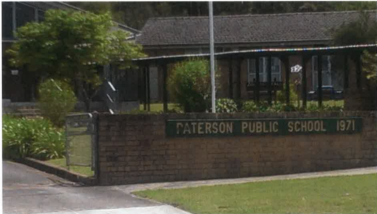
Paterson Public School – north-west from subject property on opposite side of Webbers Creek Road
