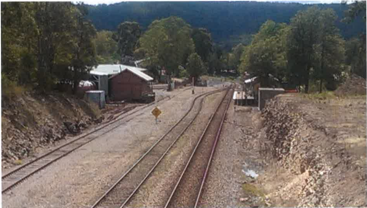
Paterson Railway Station looking North from pedestrian footbridge connecting eastern and western portions of Paterson village
